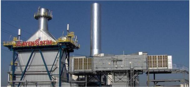
Picture .1- Sample Application of a Combustion Turbine Inlet Air Cooling Unit
