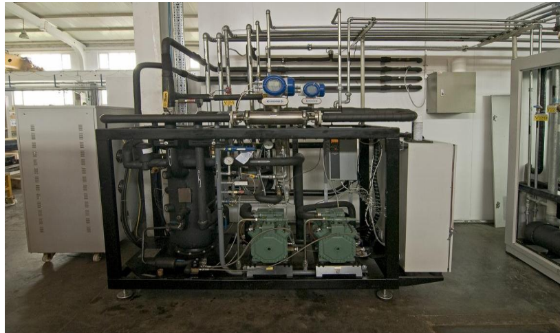
Figure 24. CO 2 refrigerant preparation unit [27]
